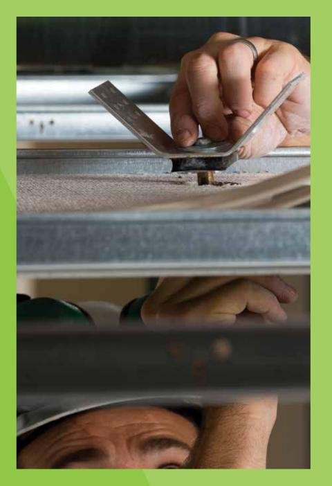
3/ Create 9mm hole and bolt TRACKLOK<sup>®</sup> firmly to head track using washer and bolt provided.
