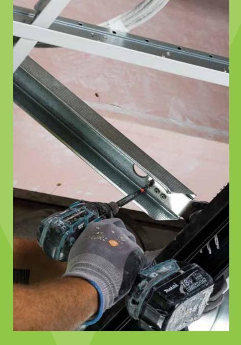
8/ Connect bracing material to TRACKLOK<sup>®</sup> fly brace with #10-gauge wafer tek screws.
