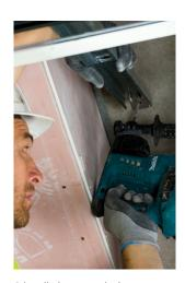
**9/** Drill clearance hole into structure over.
