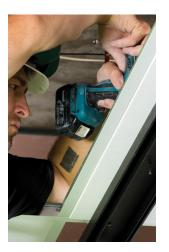
2/ Create 30mm to 40mm clearance hole in ceiling tile with holesaw (pilot bit marks centre point on head track).
