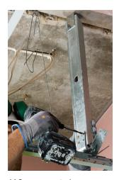
**6/** Connect vertical arm to GRIDLOK® unit and rotate to avoid service clashes.
