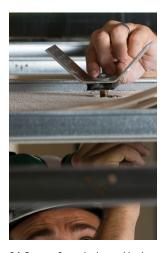
3/ Create 9mm hole and bolt TRACKLOK® firmly to head track using washer and bolt provided.
