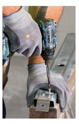
7/ Connect bracing material to TRACKLOK® top connector with #10-gauge wafer tek screws.
