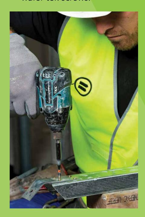
**5/** Attach 45° top connector to cut stud.
