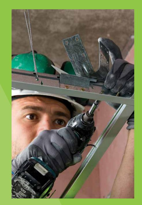
1/ Place GRIDLOK® in position specified on ceiling grid main runner or top cross rail and fix with #10-gauge wafer tek screws.
