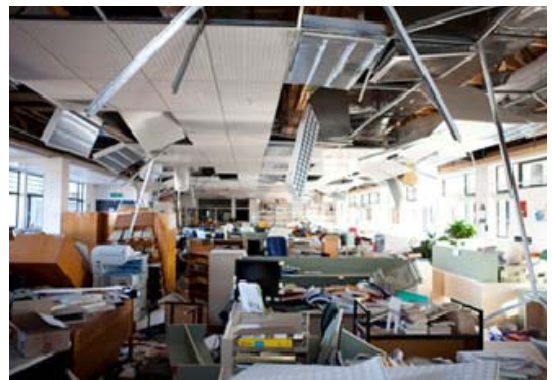
Figure 68: Damage to ceiling tile from an unrestrained fire protection system.
