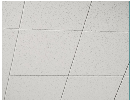
Figure 12: Concealed grid.
